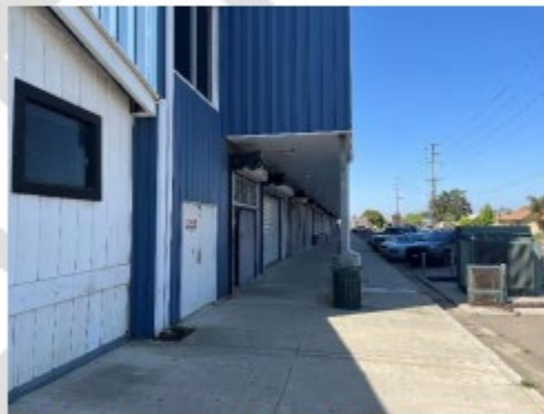
North elevation & breezeway, Building C
