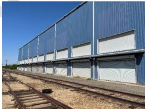
West side of Building C
