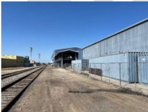
West side of Building A
