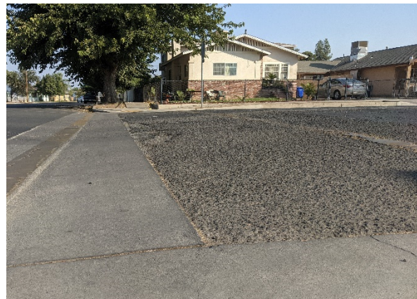
Left: Alligator cracking and raveling in asphalt. (8/31/21) Right: Raveling and potholes at Homassell & Hermosa Intersection (8/31/21)
