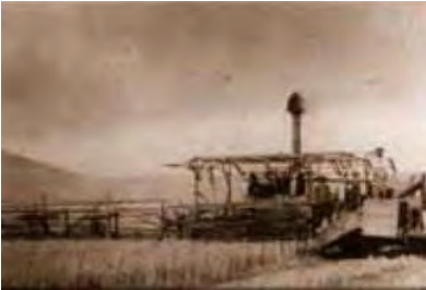
G.S. Berry and the first self-propelled harvester around 1885. It used the stalks of the wheat for fuel. The chance of fire was great as the sparks could ignite the entire fields of grain before it was harvested.
