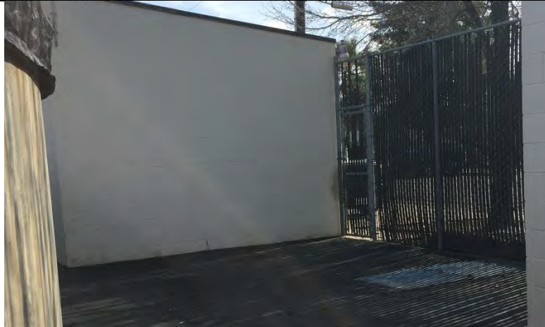
Figure 4. Future Chemical Enclosure Location
